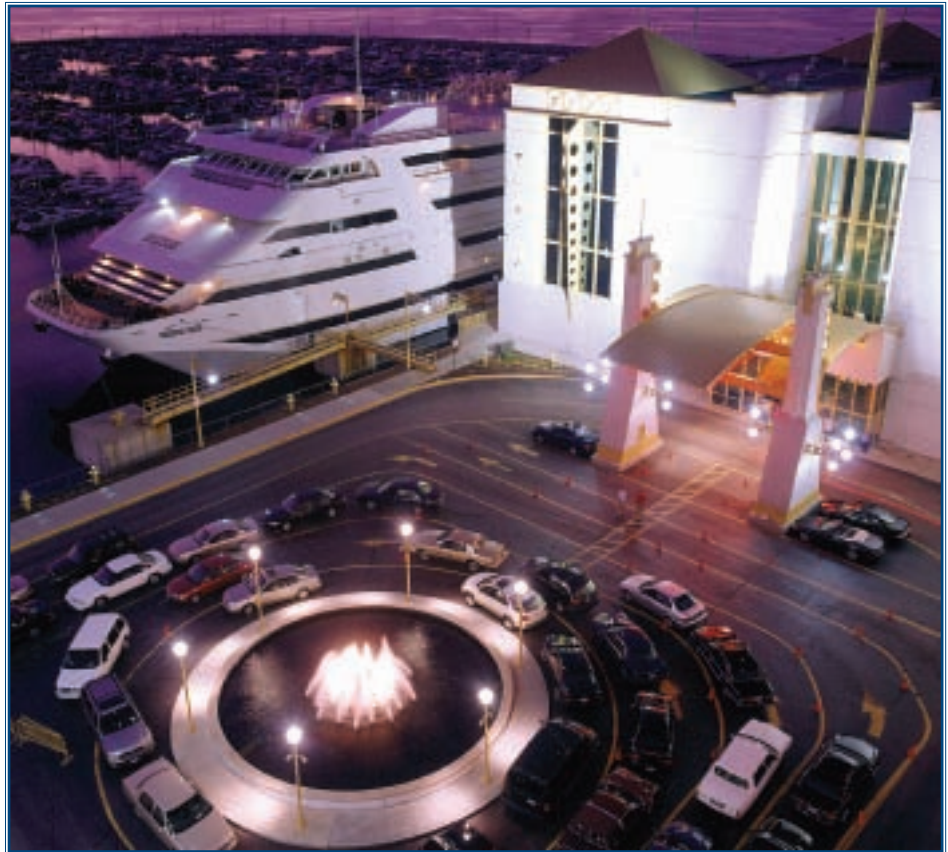
Even at night, the Horseshoe Casino never sleeps. This creates unique challenges for cleaning the over 100,000 square feet of carpet that covers the casino floors and the adjacent entrance pavilion.
