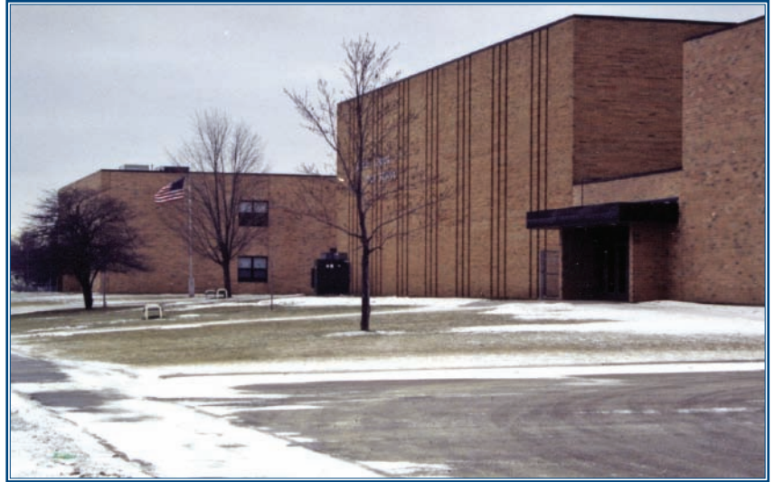
Tomah High School is one of nine schools in the district where half a million square feet of carpet is maintained with the HOST® Dry Extraction Carpet Cleaning System.
